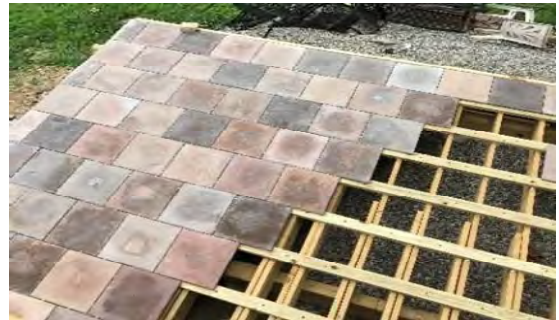
OVER CONCRETE INSTALL
